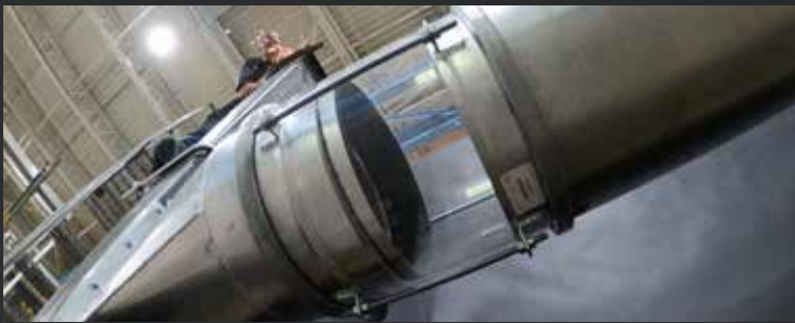
WITH AN INTEGRATED SPARK TRAP
