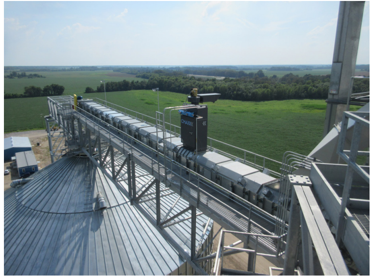
A CMAXX Spot Filter controls dust at a grain facility.
