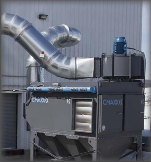
**This system is protected by the IDA DeltaMAXX Technology. Return air is now isolated from a flame front.**
